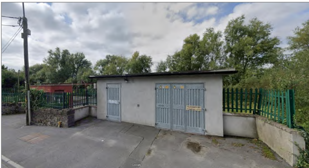
Plate 4. Kilkenny Road Pumping Station showing small red-brick building and cement building
